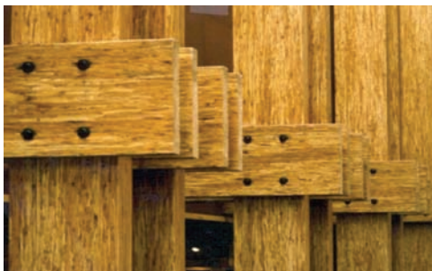
Figure 2. Bolted connections used in heavy timber construction
