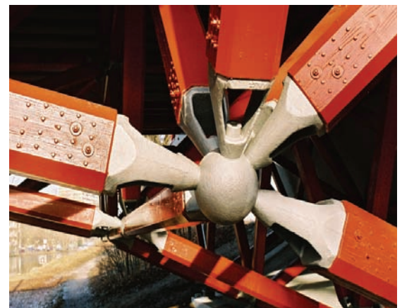
Figure 3. Steel dowel connection
