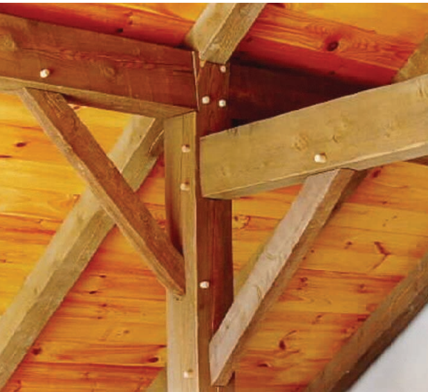
Figure 1. Timber frame using connections with wooden pegs
