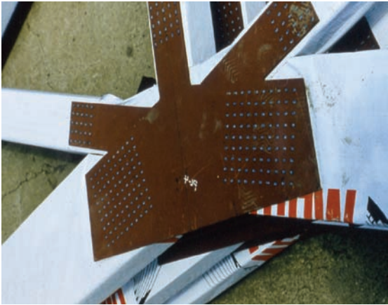
Figure 4. Glulam rivets used in heavy timber construction
