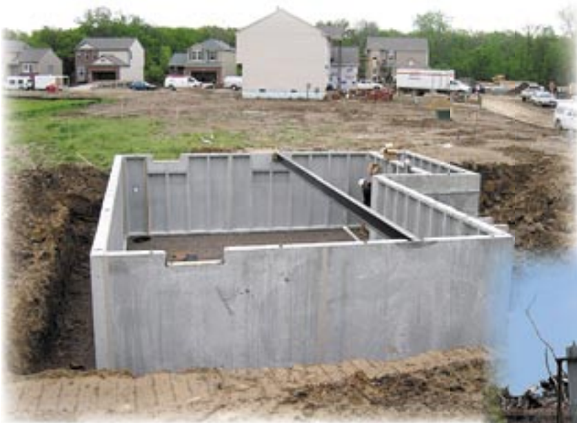
Prefabrication is also making its way through concrete foundations
