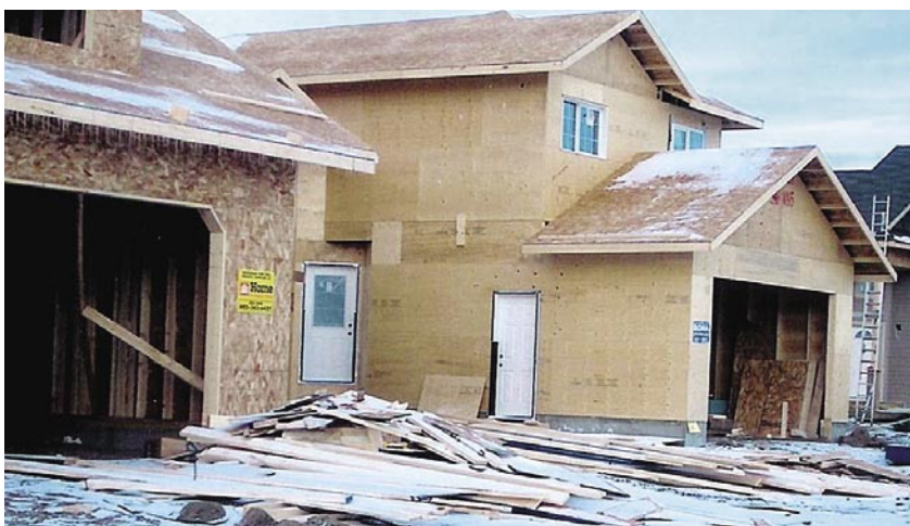
Building houses on-site creates considerable waste
